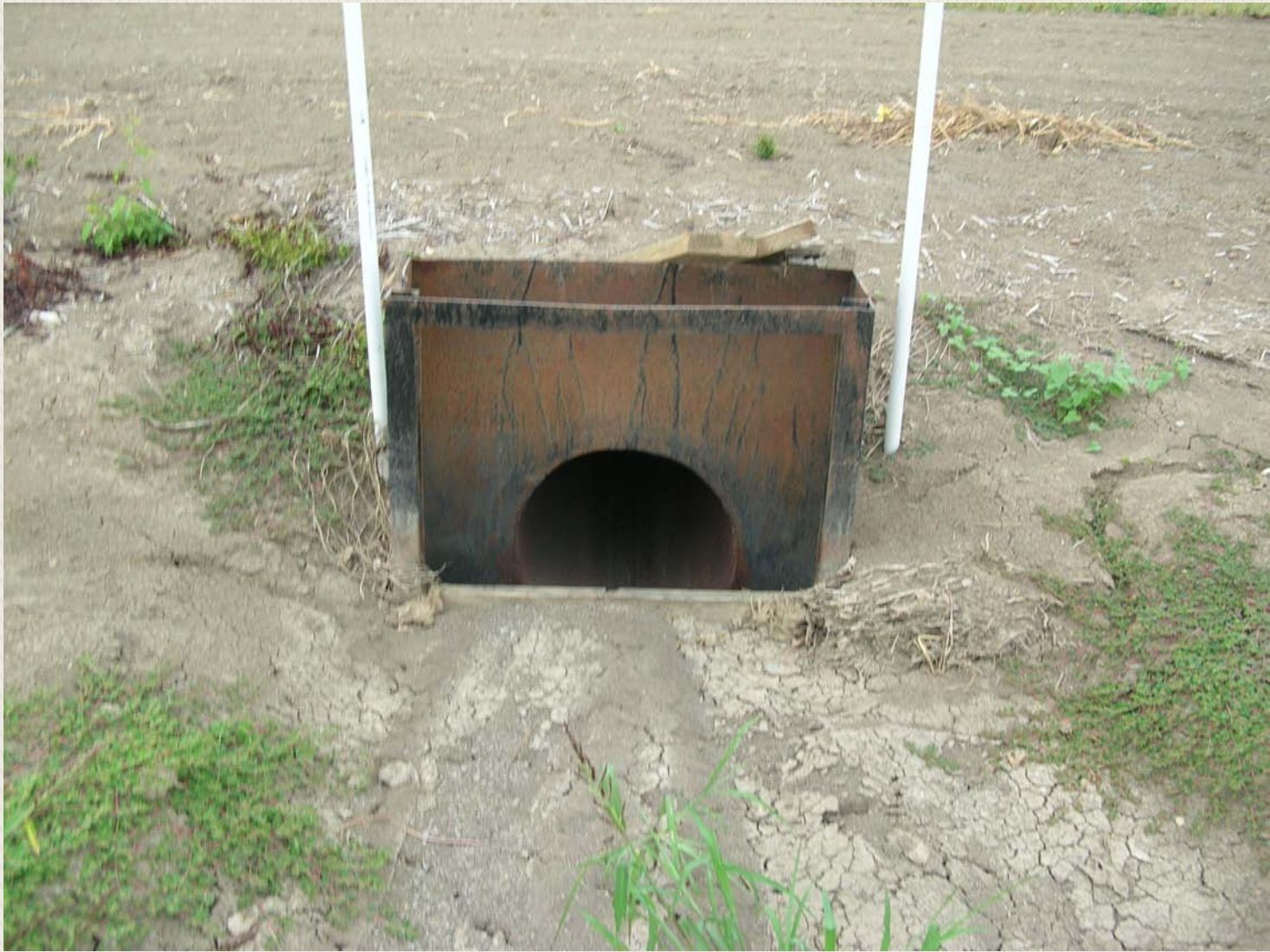
Water Control Structure
