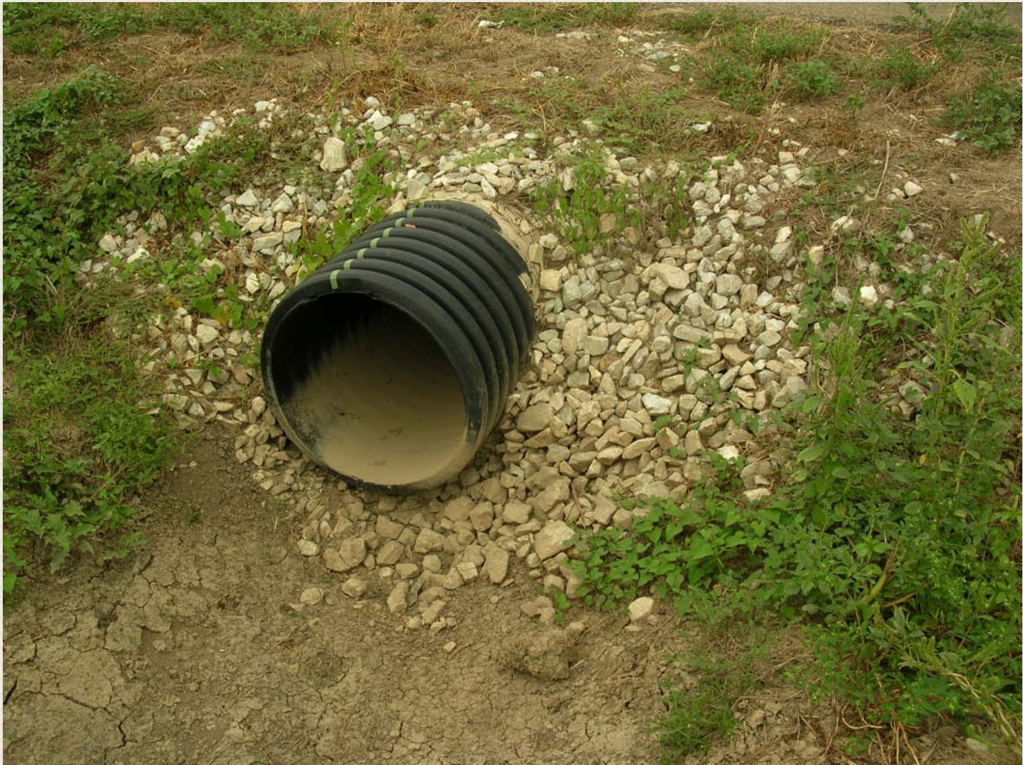
Drop pipe installed with stabilization rocks
